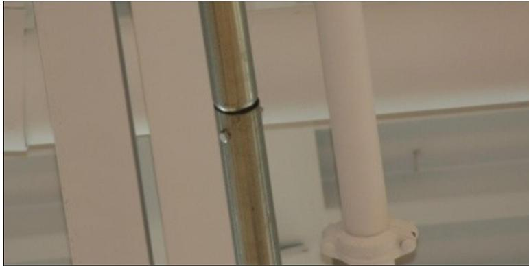
Figure 17: Typical Drive Pipe Splice Assembly
